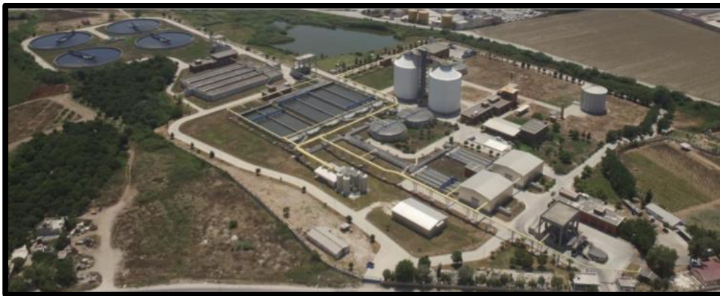
Figure 8-10. Yüreğir WWTP (Source: Official website of Adana ASKI)
