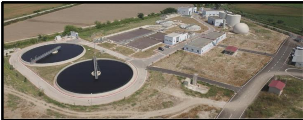
Figure 8-11. Aerial view of the Ceyhan WWTP (Source: Official website of Adana ASKI)
