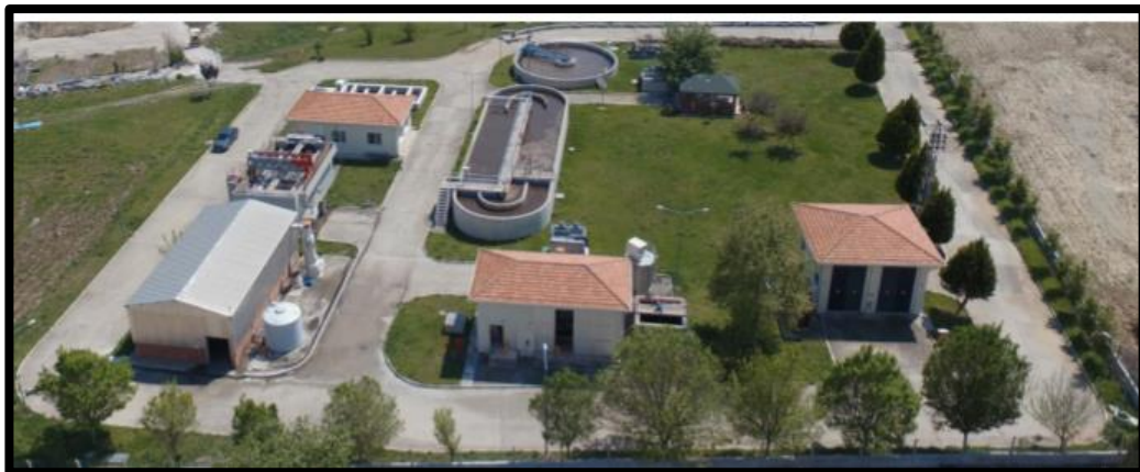
Figure 8-12. Aerial view of the Karaisalı WWTP (Source: Official website of Adana ASKI)
